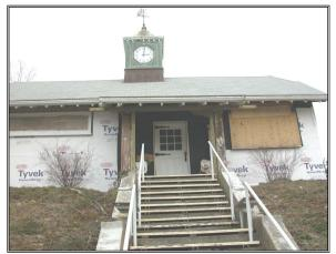
The old siding has been removed, windows are being repaired, and there are warning signs posted on the front steps leading up to the Cobb Library - renovations have begun!
